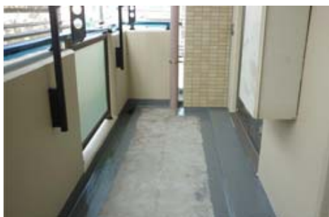
[バルコニー施工前]
